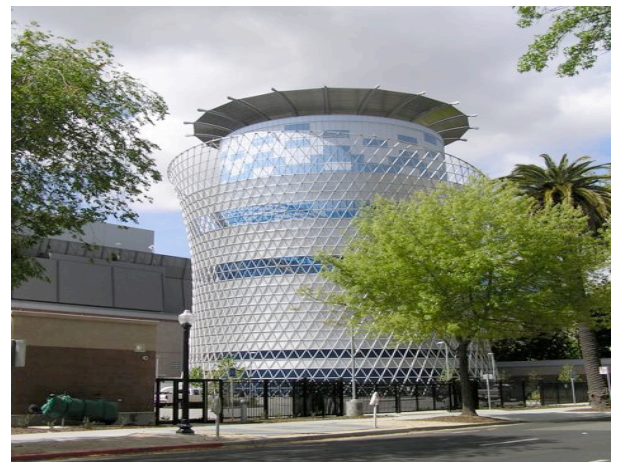
DGS Central Plant
