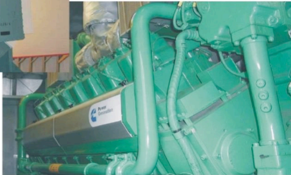
Below: 16-cylinder 1,100 kW reciprocating engine from Cummins
