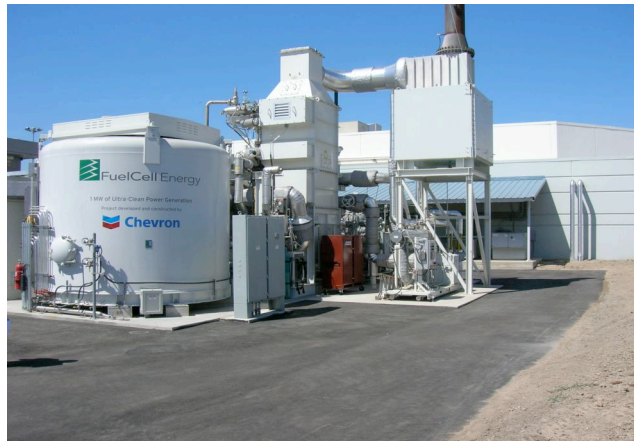
1 MW single direct fuel cell module at the Santa Rita jail
