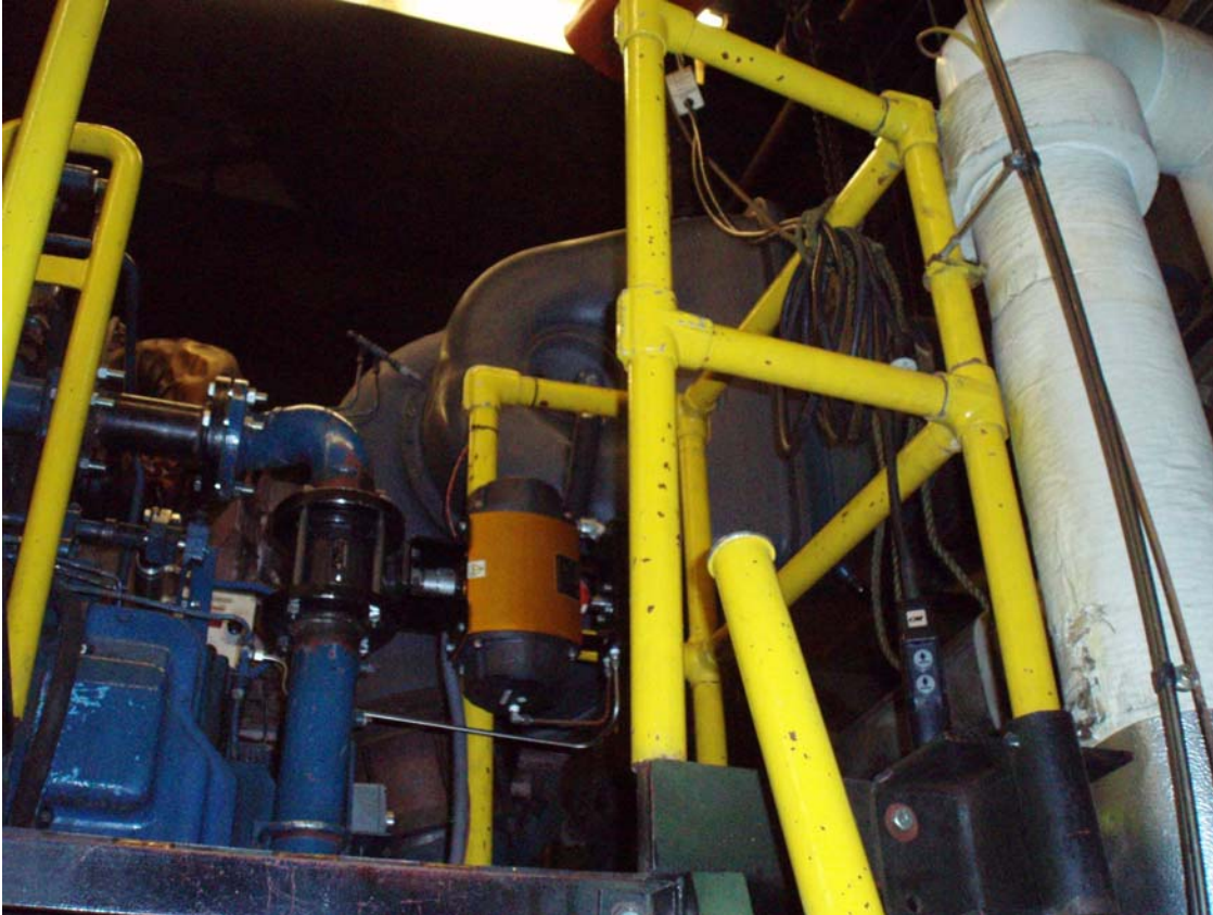
Figure 6: Exhaust routing for the turbocharger
