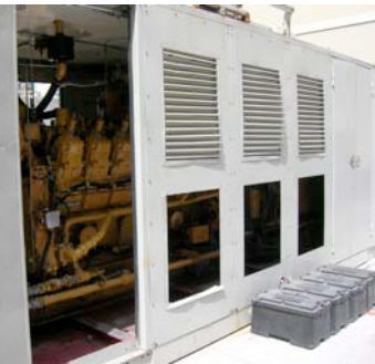
Pictured: Caterpillar reciprocating engine generator and hot water loop
