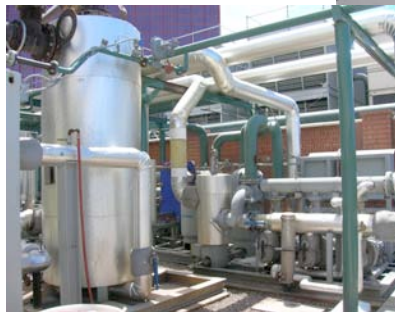
Pictured: Caterpillar reciprocating engine generator and hot water loop
